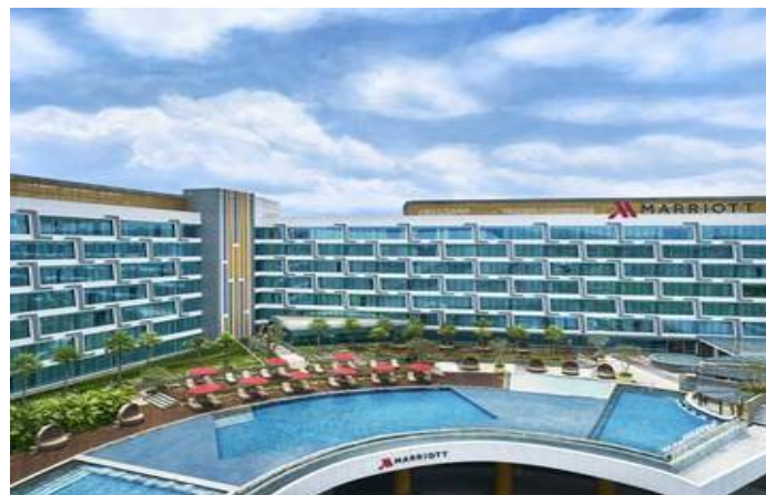
Exterior Swimming Pool
