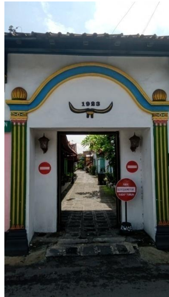
Pintu masuk Between Two Gates Sumber : Dokumen pribadi
