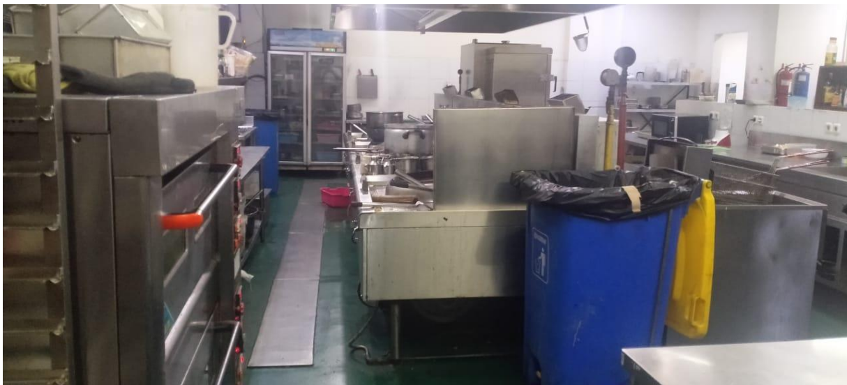
Gb. 4 Ruang Hot Kitchen
