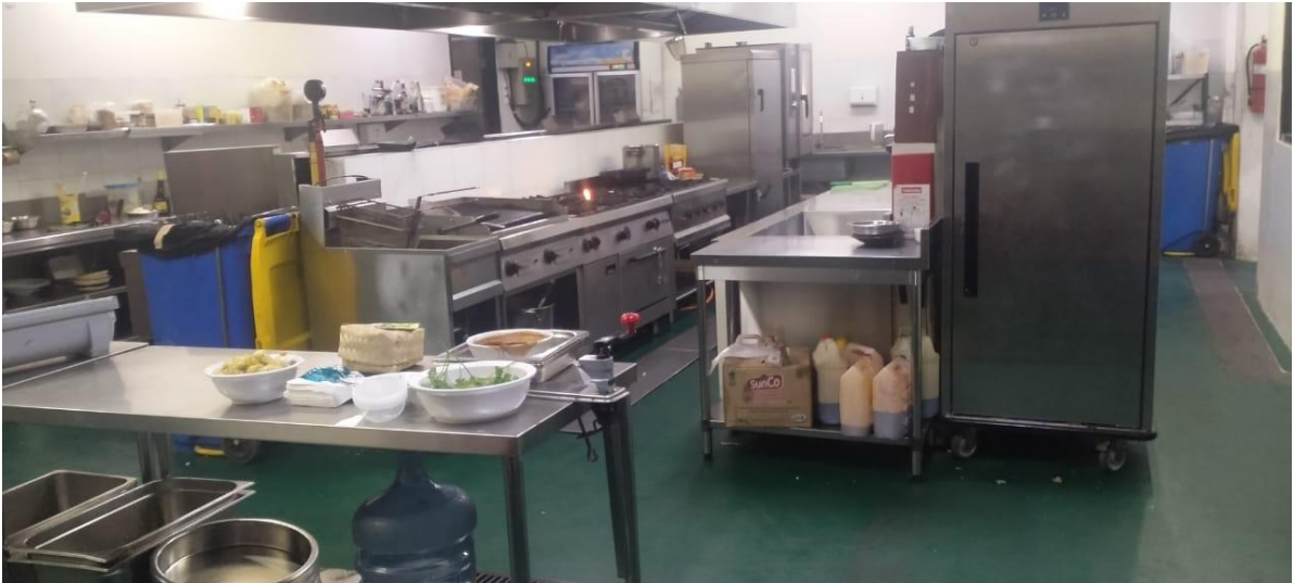
Gb. 5 Ruang Hot Kitchen
